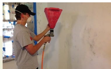
David applying texture to sheet rock walls.
